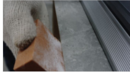
5.4.3 Rub the cuts with abrasive block to smoothen the rough edge
