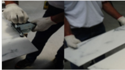
5.1.5 Apply the pliers to split the cuts and apply enough and even pressure
