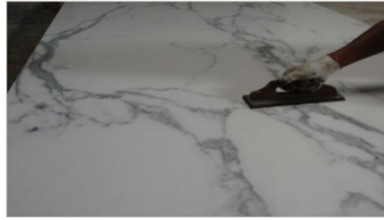
4.1.5 Tap rubber to compact the adhesive layer
