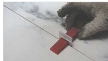
4.2.6 Put leveler at each linear meter of Quadra
