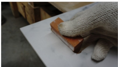
5.2.4 Rub the cuts with abrasive block to smoothen the rough edge
