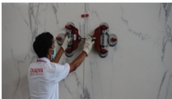
4.1.7 Use seam closer to adjust the gap of Quadra slabs
