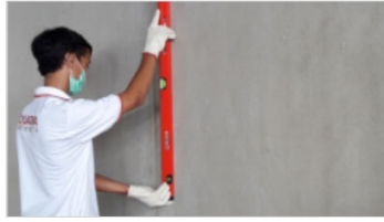
4.1.2 Make sure the wall and the back of Quadra is clean and flat
