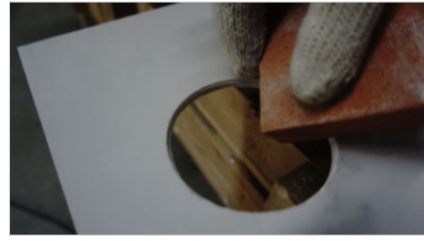
5.3.3 Rub the cuts with abrasive block to smoothen the rough edge
