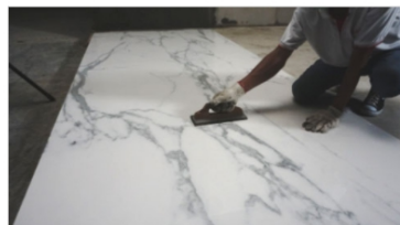
4.2.5 Tap rubber to compact the adhesive layer
