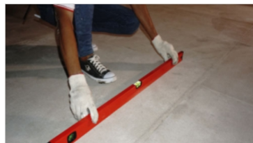
4.2.2 Make sure the wall and the back of Quadra is clean and flat
