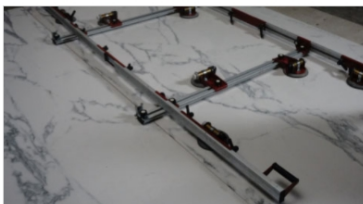
4.2.4 Lay Quadra on the adhesive bed
