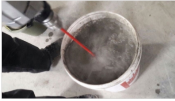
4.1.1 Mixed water and adhesive proportionally and use only adhesive class C2TES1 to get the best result
