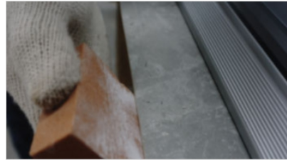
5.1.6 Rub the cuts with abrasive block to smoothen the rough edge
