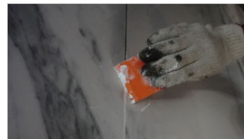
4.1.9 Apply the grout onto the wall
