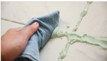
4.1.10 Clean the grout waste
