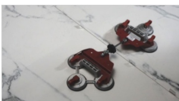
4.2.7 Use seam closer to adjust the gap of Quadra slabs
